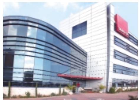
Taro's new facilities in Haifa, Israel (shown here) and Toronto, Canada put additional state-of-the-art equipment in the hands of Taro scientists.
