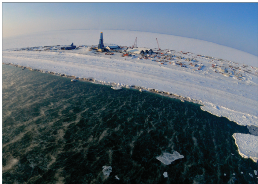
On Sakhalin Island, the Yastreb drilling rig has been moved from Chayvo to Odoptu and is now drilling extended-reach development wells into this offshore field from the onshore location pictured above.
