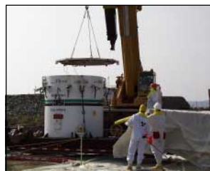
Top left: The carbon steel, lead shielded 10-160B is more than seven feet tall and over six feet in diameter and weighs 72,000 pounds with its contents.
