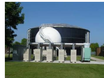
Waste Water Plants
