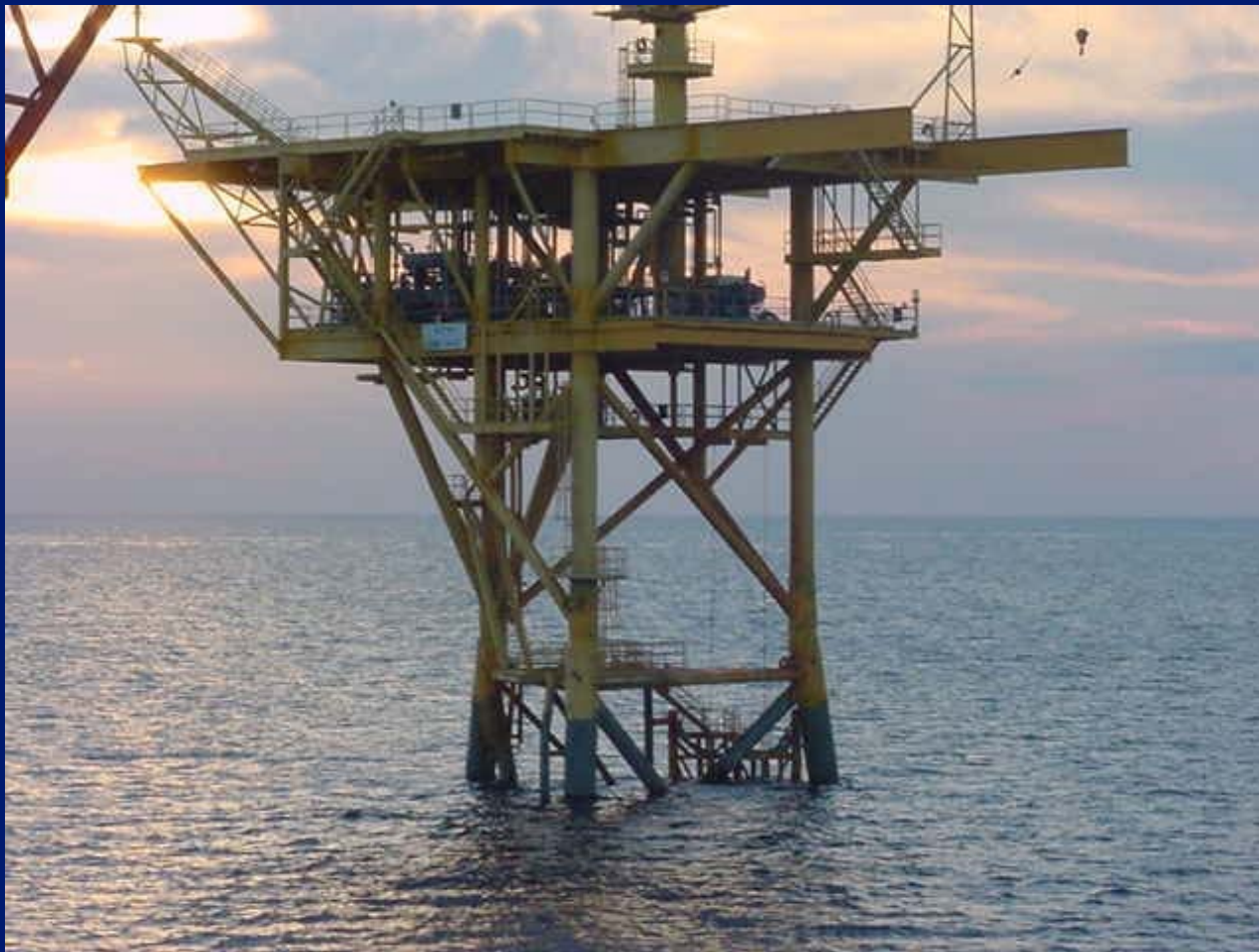
Platform & deck installation
