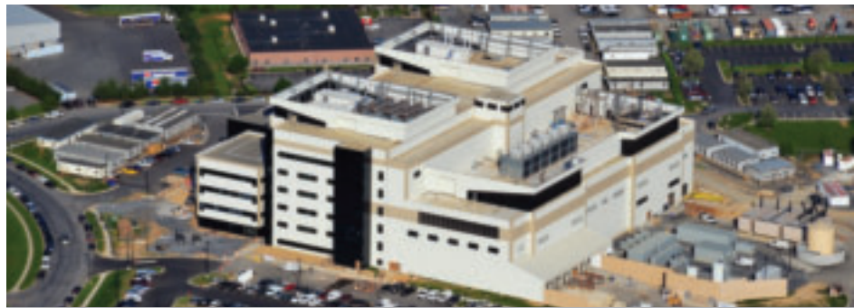
Fluor is providing construction management and commissioning services for MedImmune's 300,000-square-foot manufacturing facility in Frederick, Maryland, to produce its high-value biological products.
