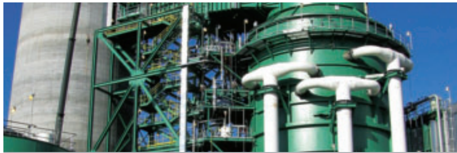
Fluor is providing EPC services to SCE&G, the principal subsidiary of SCANA Corporation, for the installation and commissioning of Wet Flue Gas Desulfurization (WFGD) systems at the Wateree and Williams stations located in South Carolina. Upon completion, the WFGD systems will reduce sulfur dioxide (SO 2 ) emissions by over 95 percent.
