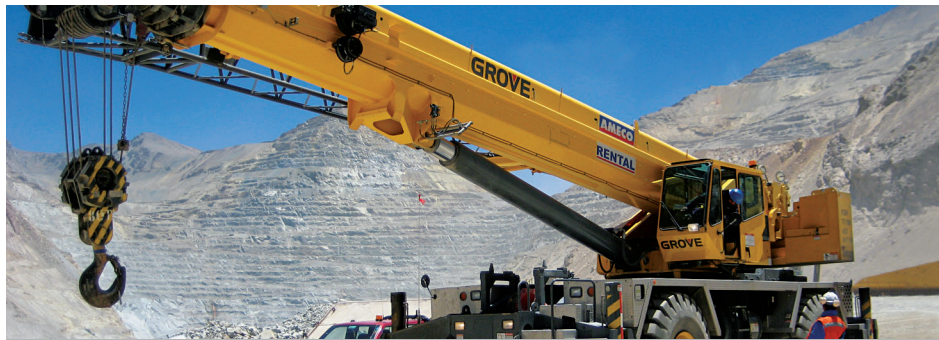
Fluor's equipment subsidiary, AMECO®, provides a fleet of fully operated and maintained cranes and earth-moving equipment to support Minera Los Pelambres' 339,000-ton-per-year copper mine in Chile.
