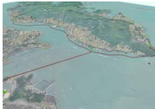
Hong Kong Harbour Area Treatment Scheme Hong Kong, China
