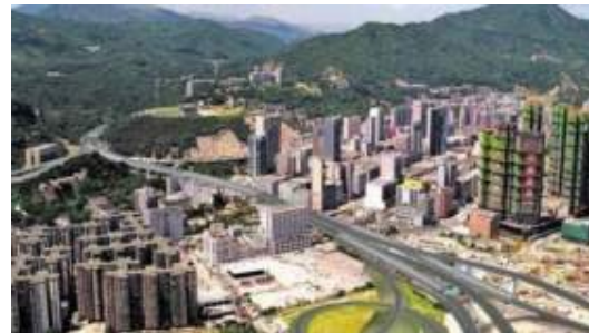
Route 8 Expressway Hong Kong, China
