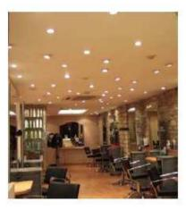
Salon lit solely with recessed dichroic halogen fittings. Ceiling looks cluttered and unorganised. The space also is very warm due to the heat of the lamps. Solely downward distribution of light does not light vertical surfaces (peoples faces) well, giving harsh shadows and being very unflattering.
