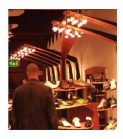
Store solely lit with dichroic halogen lamps very inefficient lighting scheme, clustered lamps may produce scorch marks from heat thrown backwards. Excessive heat will also require additional air conditioning.
