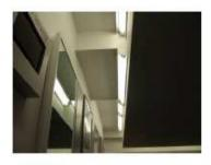
Walls are washed by angled fluorescent battens hidden in recessed pelmet detail, preventing glare from exposed battens
