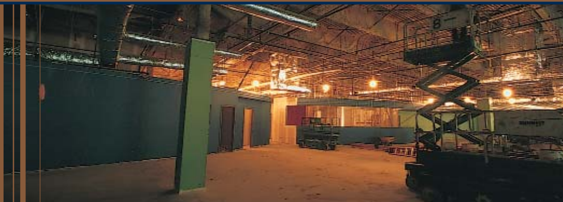
Our new Hampton, Virginia, call center under construction.
