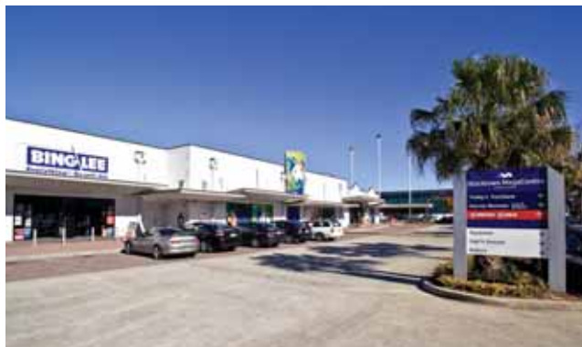
BLACKTOWN MEGA CENTRE BLACKTOWN ROAD, BLACKTOWN, NSW
