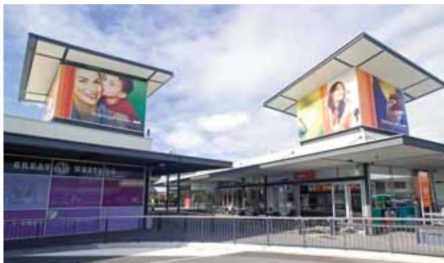
STANHOPE VILLAGE SENTRY DRIVE, STANHOPE GARDENS, NSW
