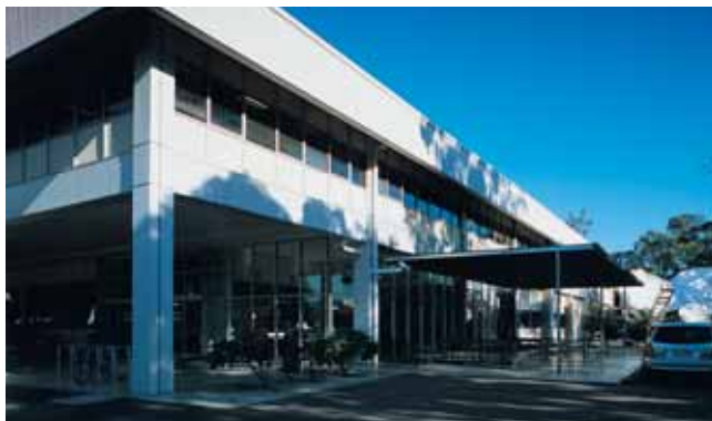
271 LANE COVE ROAD, NORTH RYDE, NSW
