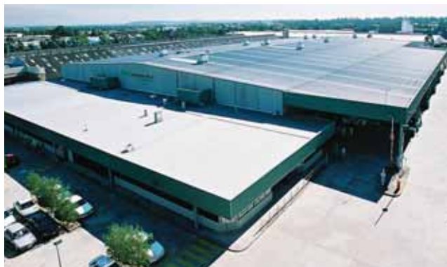
44 BILOELA STREET, VILLAWOOD, NSW
