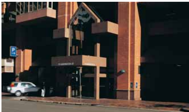
QUAY WEST CAR PARK 109 – 111 HARRINGTON STREET, SYDNEY, NSW
