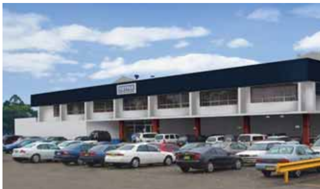
64 BILOELA STREET, VILLAWOOD, NSW
