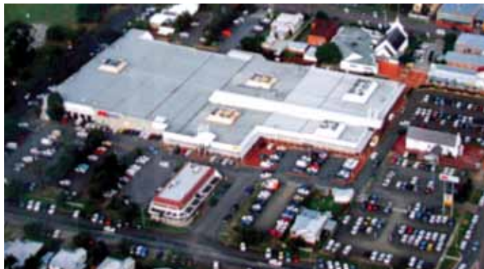
MANNING MALL, TAREE, NSW IN PROGRESS
