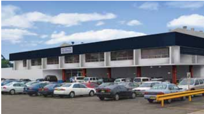
64 BILOELA STREET, VILLAWOOD, NSW
