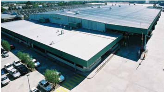
44 BILOELA STREET, VILLAWOOD, NSW
