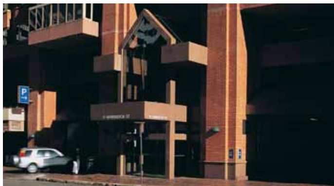
QUAY WEST CAR PARK 109 - 111 HARRINGTON STREET, SYDNEY, NSW
