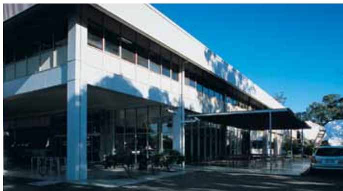
271 LANE COVE ROAD, NORTH RYDE, NSW
