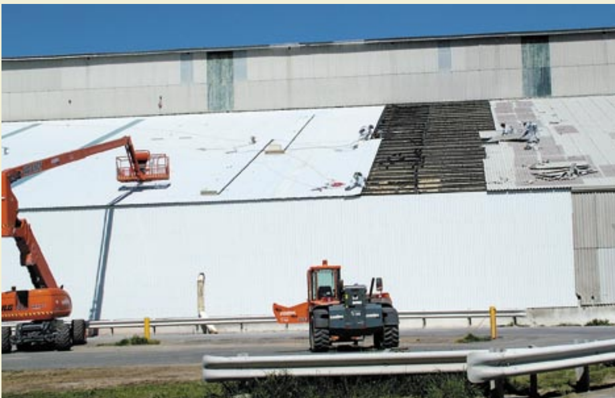
(Below) Removal of asbestos from the fertiliser sheds at Kwinana.
