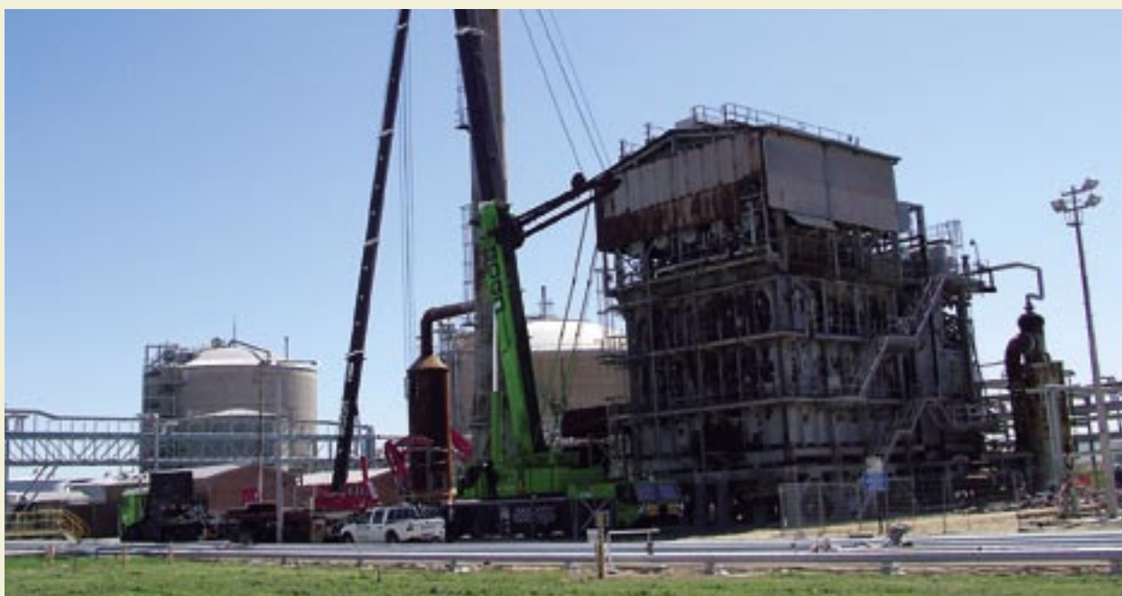
(Below) Demolition work on the decommissioned ammonia plant.
