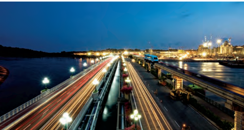
July 2009 - Completion of Sentosa's new vehicular bridge
