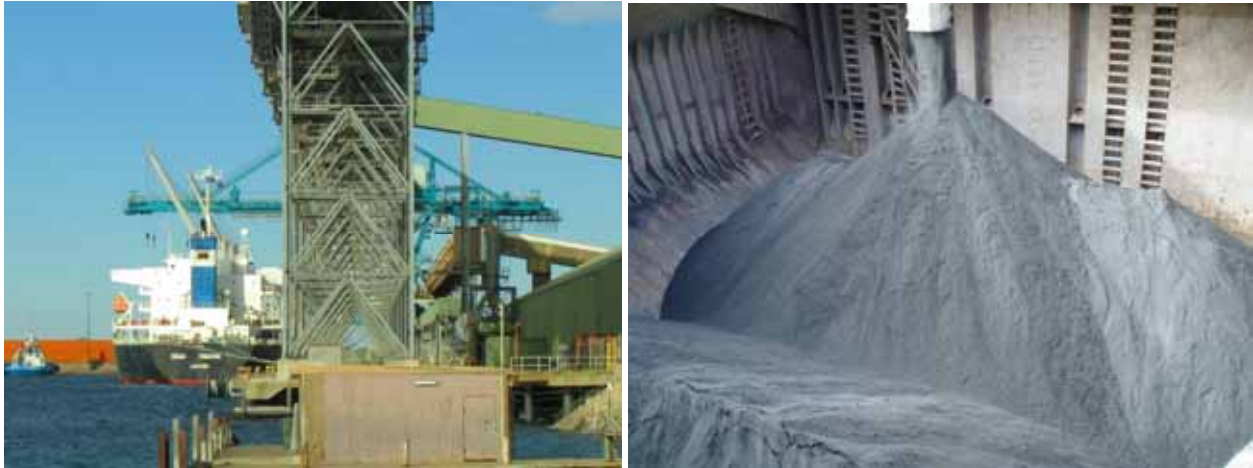
Figures 1 and 2: Loading Flying Fox nickel concentrate onto a ship at Esperance Port for export to Finland.
