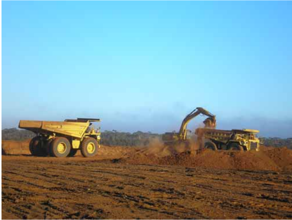
Figure 8: Constructing evaporation pond for dewatering Diggers South mine.
