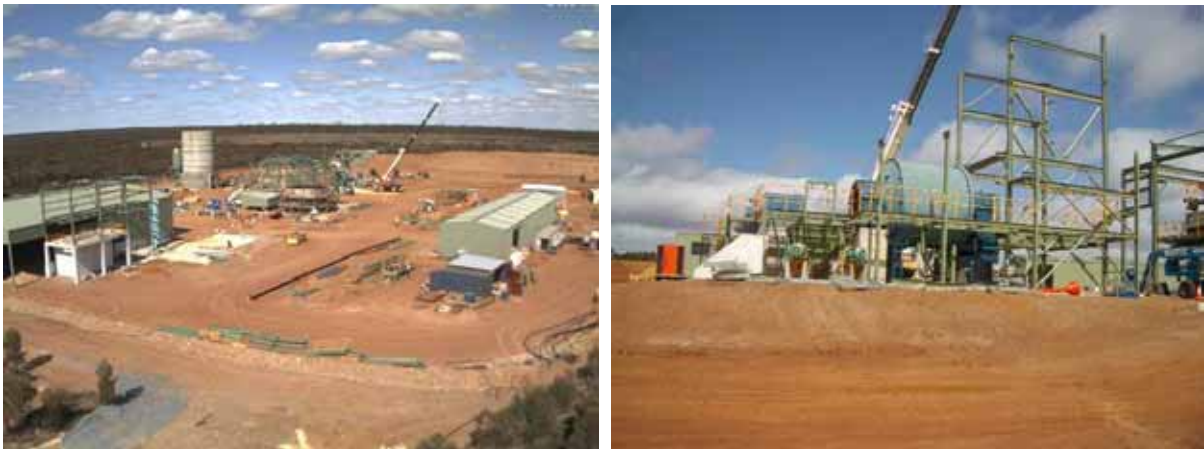
Figures 9 and 10: Cosmic Boy Concentrator Plant. Figure 9 shows the coarse ore bin on LHS background, concentrate shed on LHS foreground, workshop/store on RHS foreground, the SAG mill to RHS of crane, flotation plant and thickener in centre and ROM pad and crusher in background. Figure 10 shows installation of the SAG mill in September.
