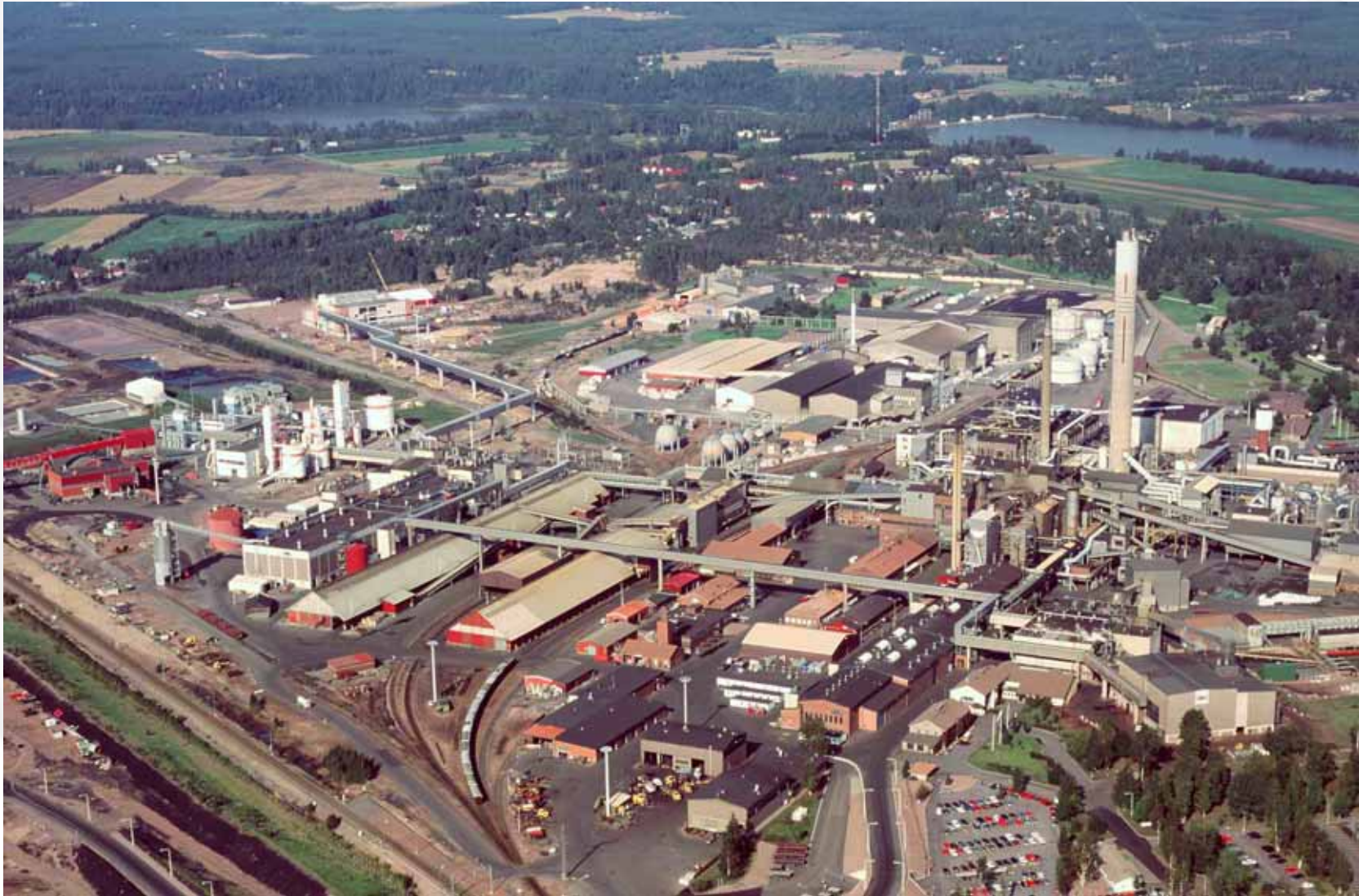
Harjavalta Nickel Smelter and Refinery, Finland
