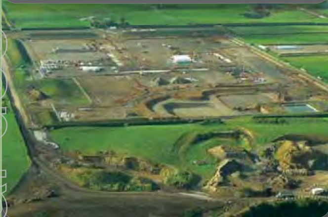
Kupe | Onshore gas plant earthworks
