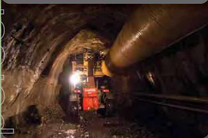
Pike River | Tunnel progress continues
