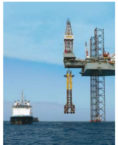
Installing the Kupe offshore platform
