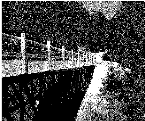
First major bridge at Pike
