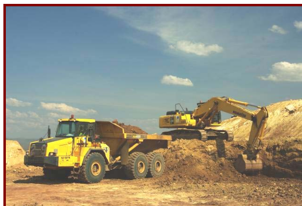
Hydraulic excavator loading diesel mine truck in Kayelekera open pit
