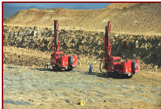
Blast hole drilling
