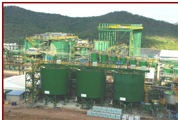
View of the Kayelekera Plant
