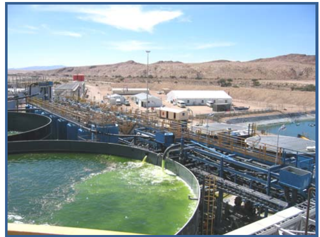
IX CIRCUIT AND SOLUTION STORAGE TANKS
