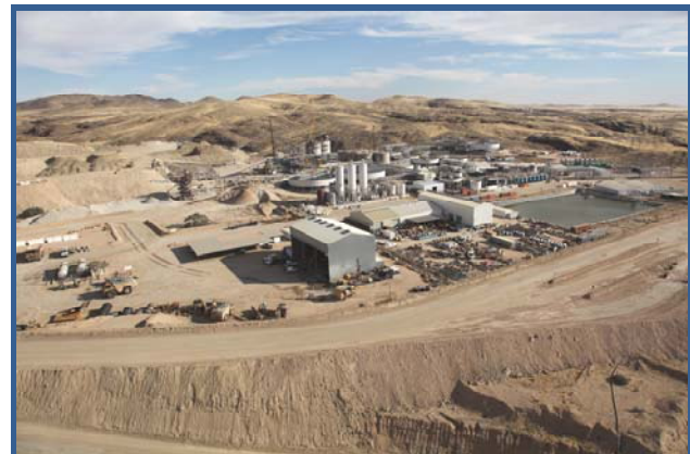
OVERALL PLANT VIEW
