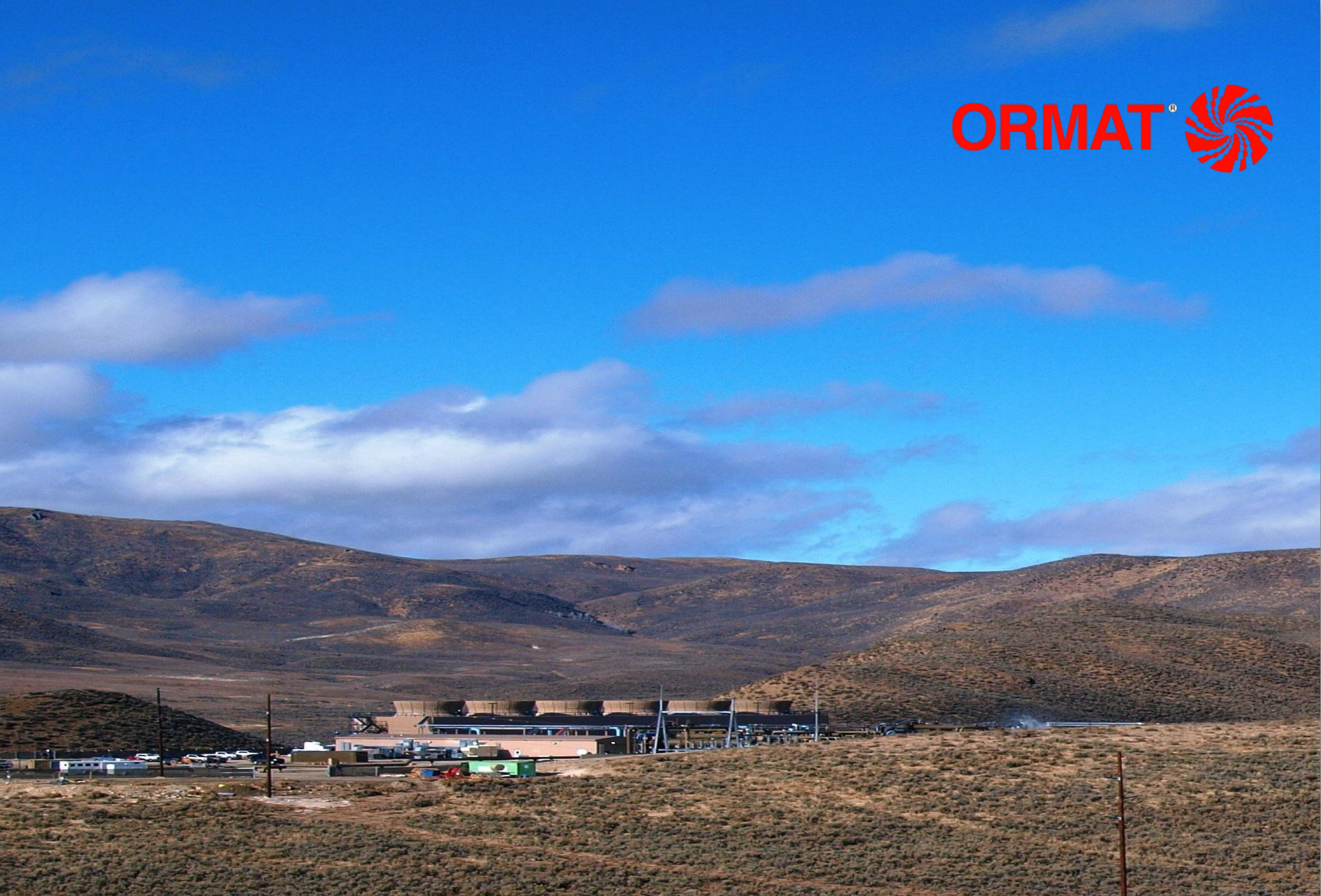
Tuscarora, Geothermal Power Plant, Nevada
