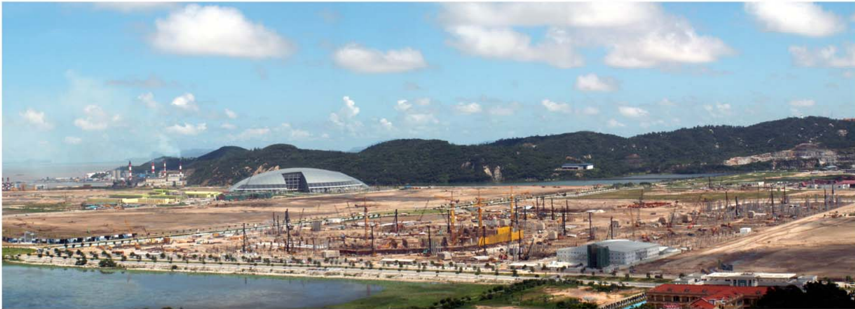
Site Progress Photo View 3 of full site
