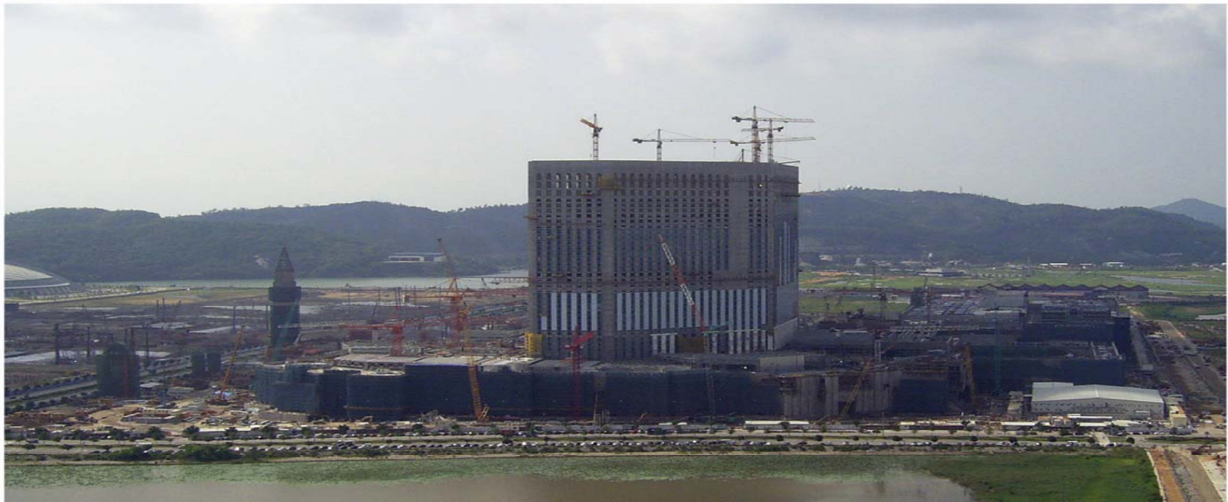
Daily site progress photo View 3 of full site
