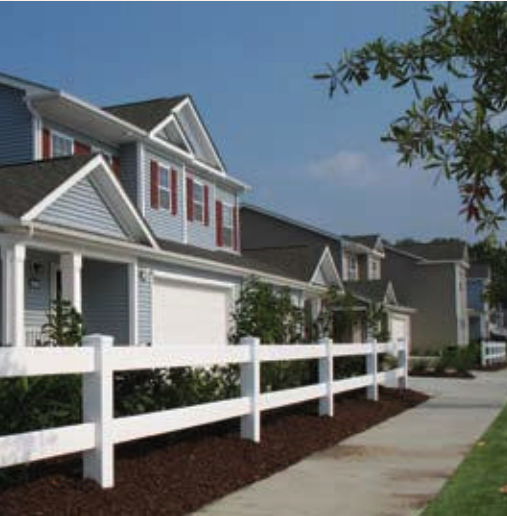
Tarawa Terrace homes at Camp Lejeune
