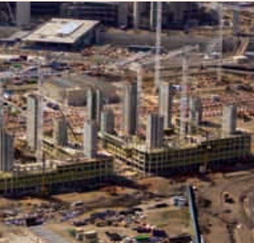
Aerial view of construction at Stratford, United Kingdom
