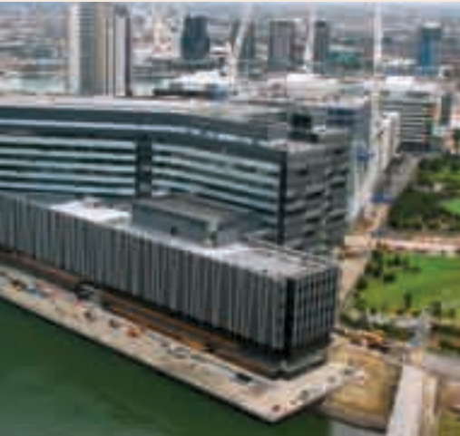
Construction of ANZ Centre, Melbourne, Australia
