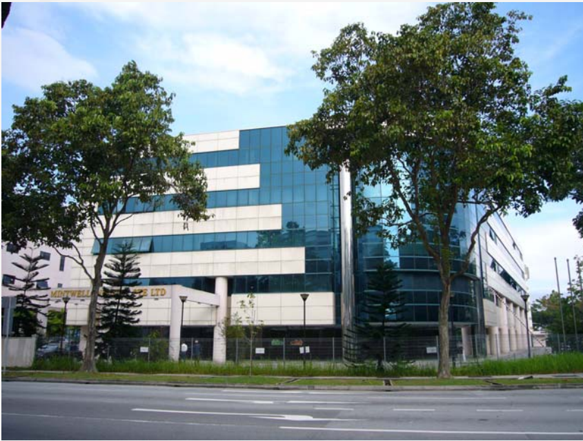
A 5-storey light industrial building with ground floor showroom.
