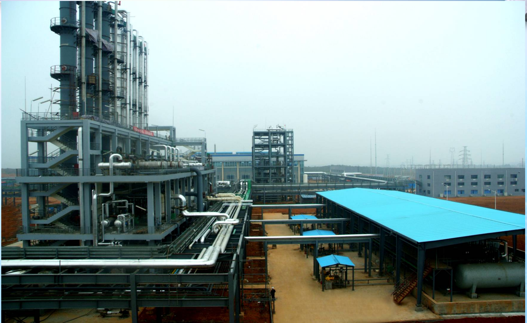
TCS Purification and Off Gas Recovery System
