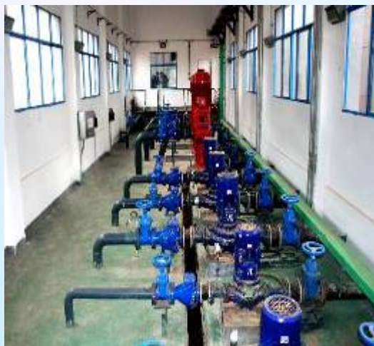
Fire water pump station
