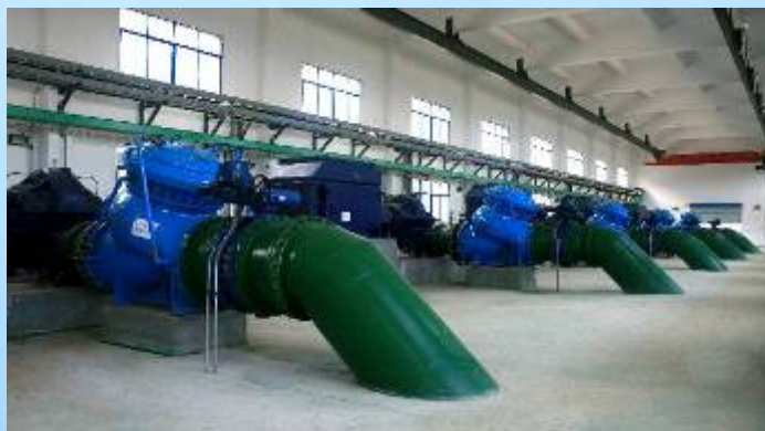
Cooling water pump station
