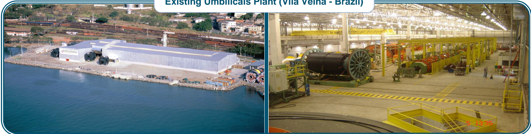
Existing Umbilicals Plant (Vila Velha - Brazil)
