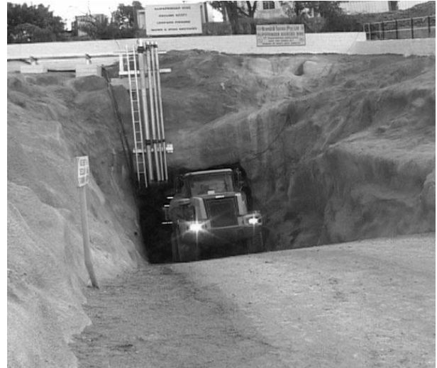
Figure 5. An example of a surface located decline entrance.
