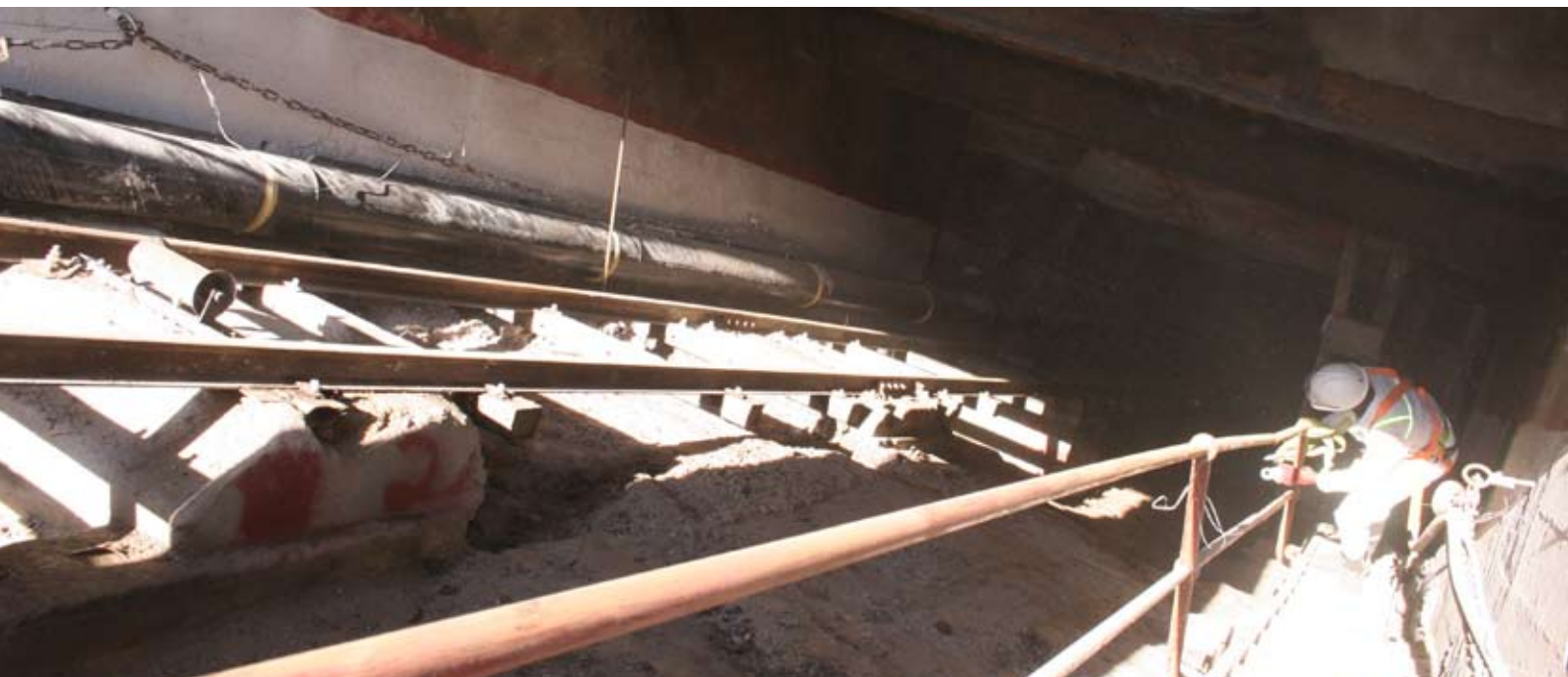
Shaft re-access program - shaft # 9
