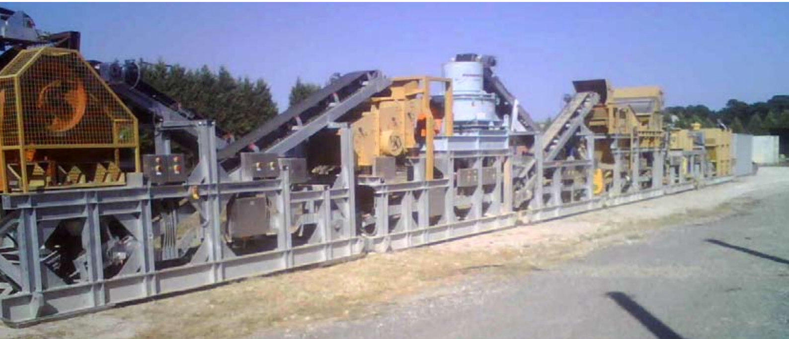
Gekko trial mining plant
