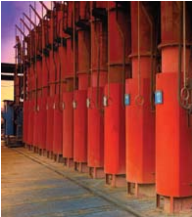
Coking Batteries, Svoboda Coking Plant
