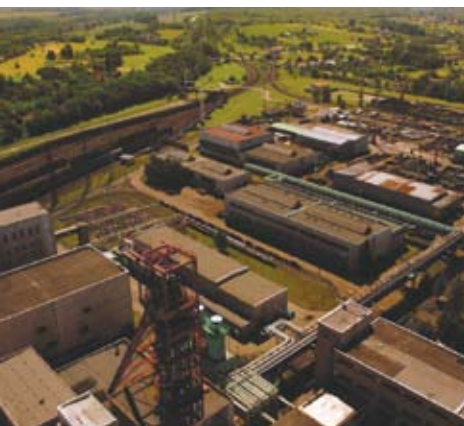
View from the hoisting tower, Darkov Mine
