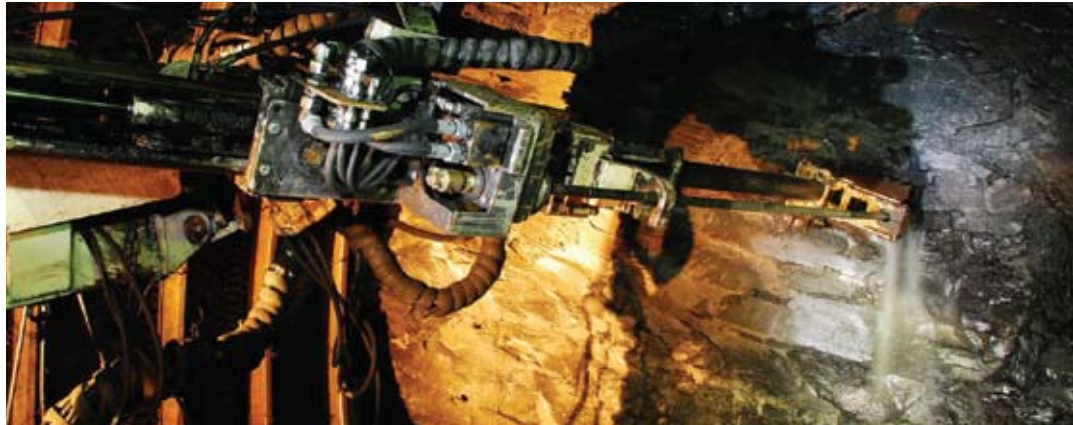
Drilling works at a development section, Staříč Site, Paskov Mine
