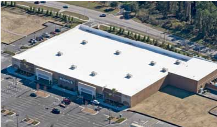
Solar reflective membranes mitigate the heat island effect in Palm Coast, Florida
