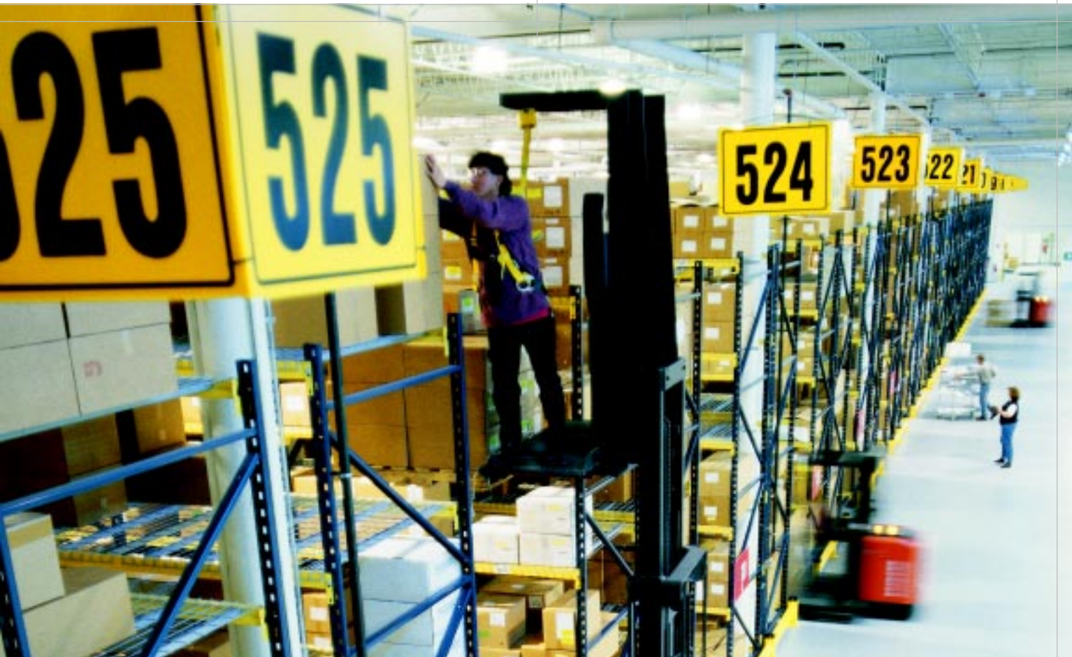
Boston Scientific's Marina Bay Customer Fulfillment Center opened in May of 1997. Located in Quincy, Massachusetts, U.S.A., the 1.3 million-square-foot facility is equipped with state-of-the-art distribution equipment, including our global information systems. By integrating inventory from all plants into one central location, we expect to realize increased U.S. distribution efficiencies of 17-20%.
