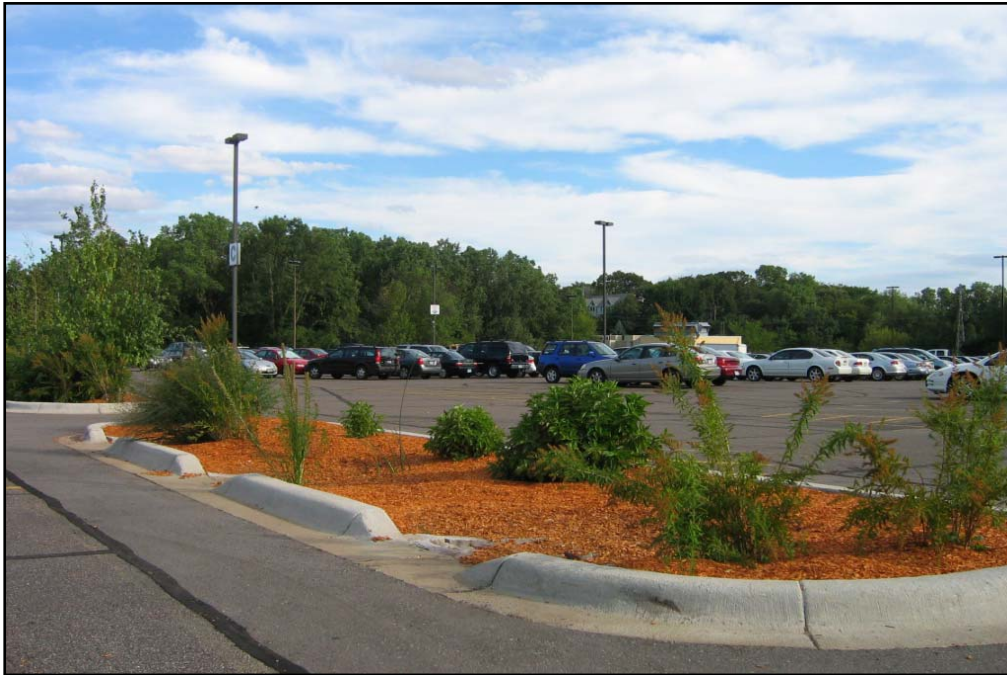
One of 16 raingardens (seepage islands) installed throughout the parking lot at Target Financial Services to capture and infiltrate stormwater runoff.
