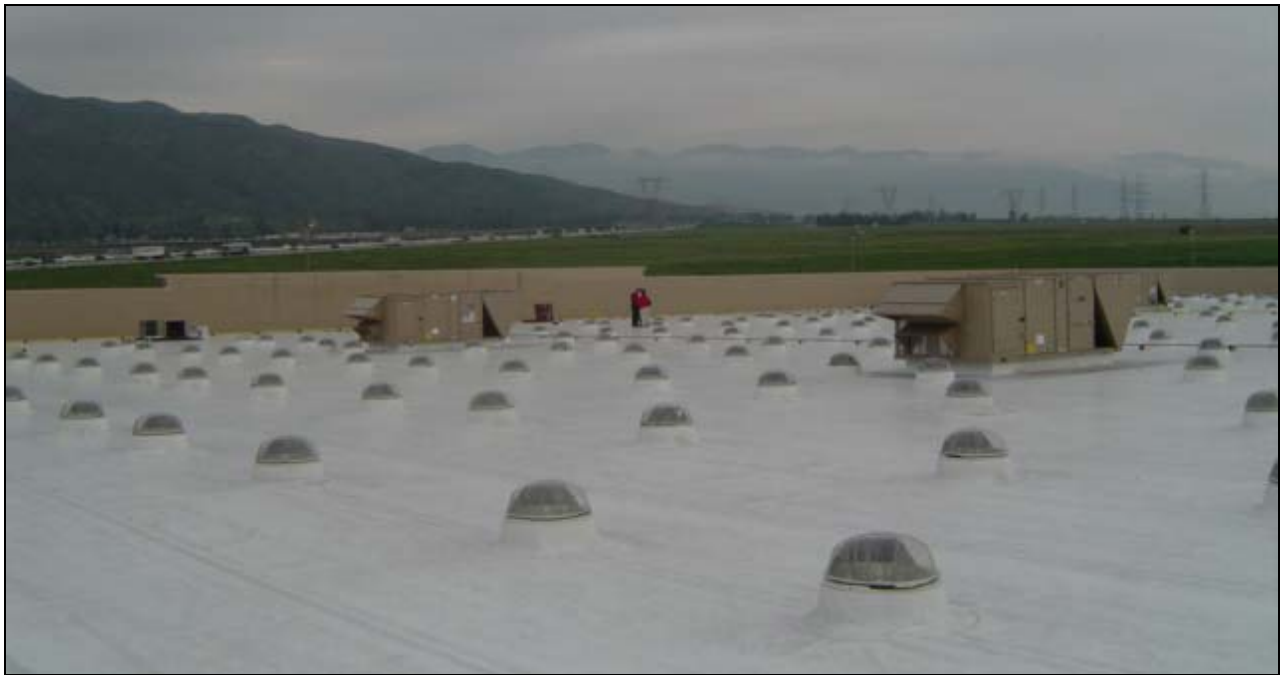
Solar tubes direct sunlight energy into the Fontana North (California) Target store.
