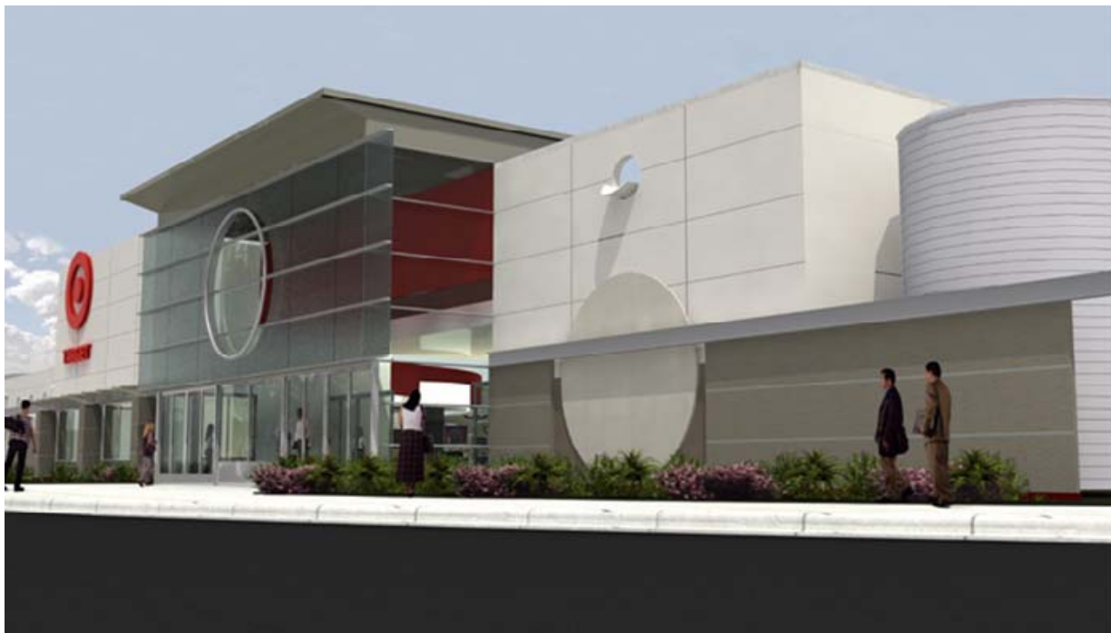
Rendering of the Allen Park, Michigan Target store, scheduled to open October 2005. Rainwater will be captured using a rooftop cistern (shown on the right).
