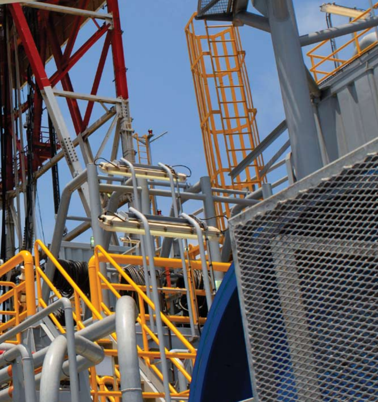
This is a look at the workings of the Ocean Endeavor, a latest-generation deepwater drilling rig.
