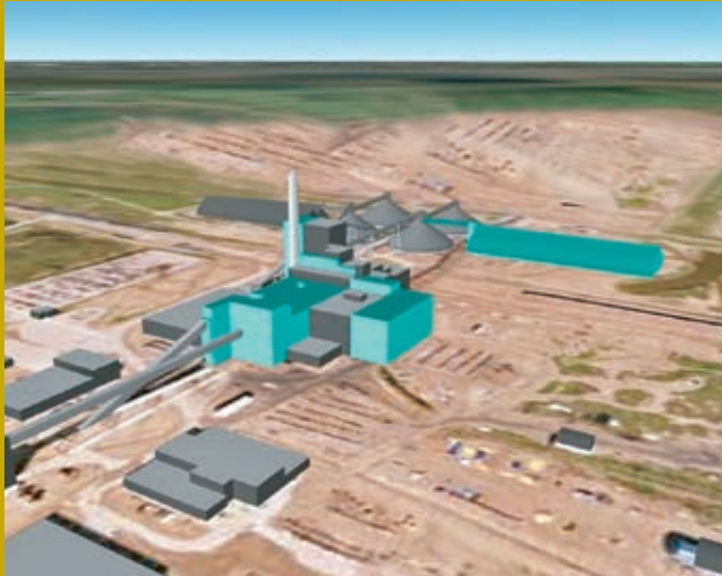
Rendering of Esterhazy expansion shows additional ground milling and product storage expansion areas (in blue), which are in addition to further underground development.
