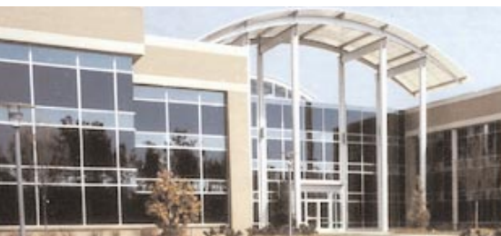
TEKELEC'S NEW R&D AND OPERATIONS CENTER IN MORRISVILLE, NORTH CAROLINA
