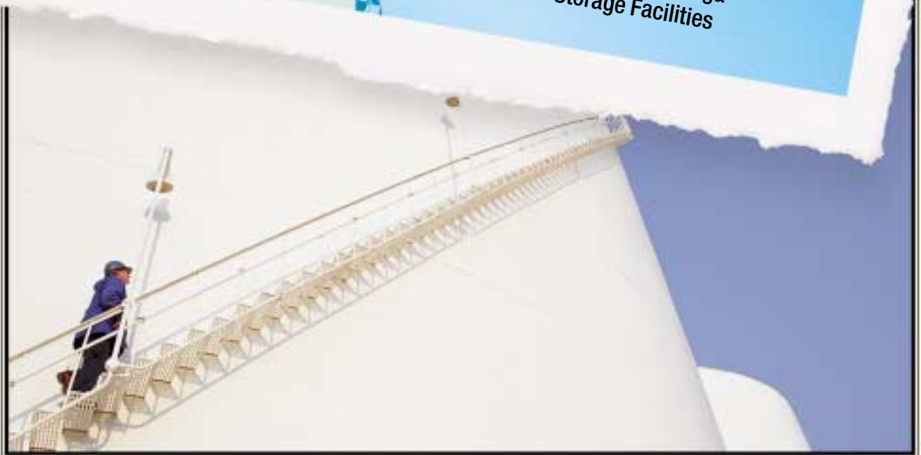
Figure 8b. LNG storage facility
