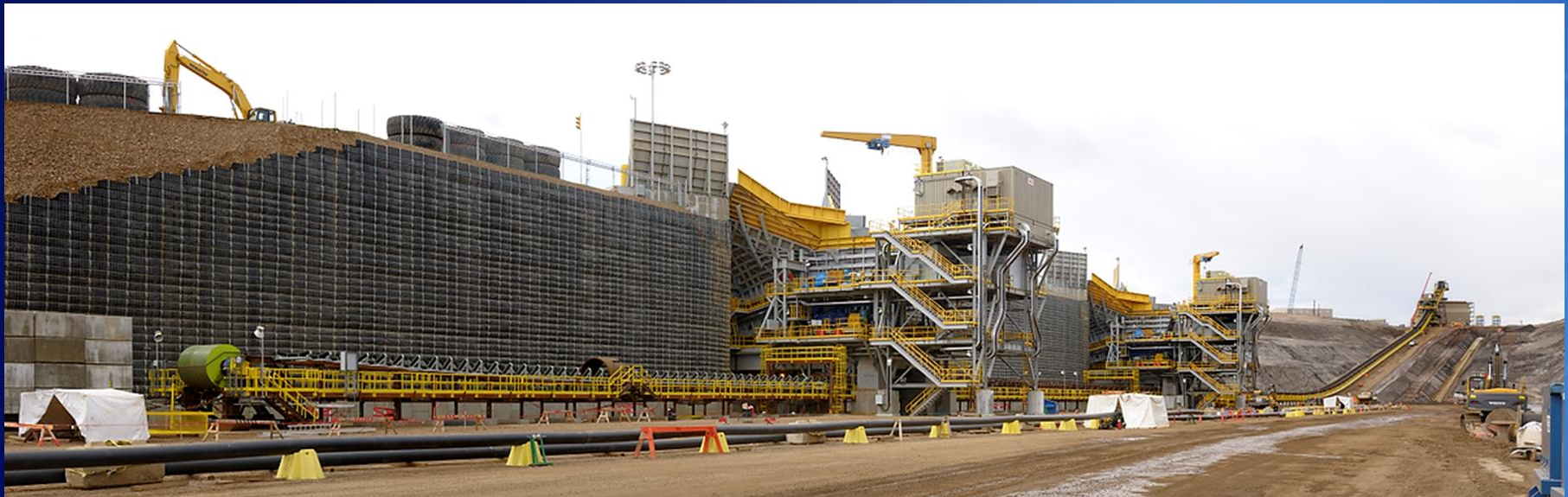
Jackpine Mine Crushers & Surge Feed Conveyor
