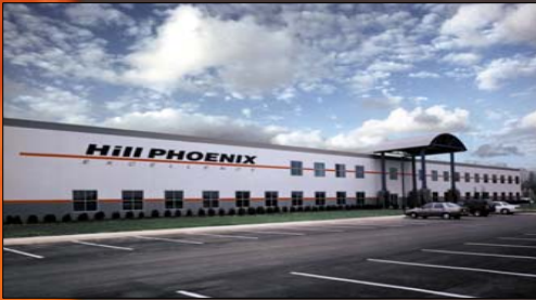
Refrigerated Case Division Plant #1 Colonial Heights, Virginia
