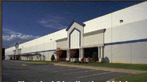
Electrical Distribution Division Conyers, Georgia
