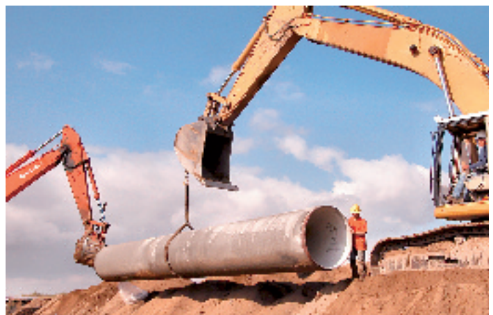
(Middle left) This 30-inch reinforced concrete pipe for the California Department of Transportation is being installed under Laguna Canyon Road near Laguna Hills, California and serves two distinct purposes: a storm drain in the wet months and a wildlife access under Laguna Canyon Road during the dry months.
