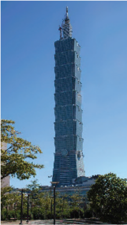
(Above) The Chinese Architectural Building Control Department chose Ameron's Steelguard® intumescent coating to protect the highest office tower in the world, called 'Building 101' located in Taipei, Taiwan.
