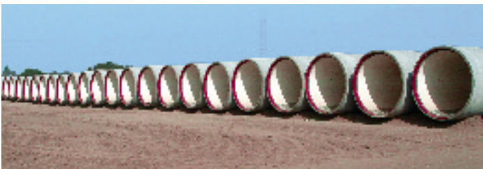
(Middle left) This 30-inch reinforced concrete pipe for the California Department of Transportation is being installed under Laguna Canyon Road near Laguna Hills, California and serves two distinct purposes: a storm drain in the wet months and a wildlife access under Laguna Canyon Road during the dry months.
