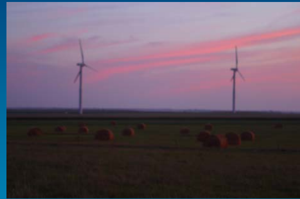
Highmore, SD GE 1.5 MW Turbines, 2003
