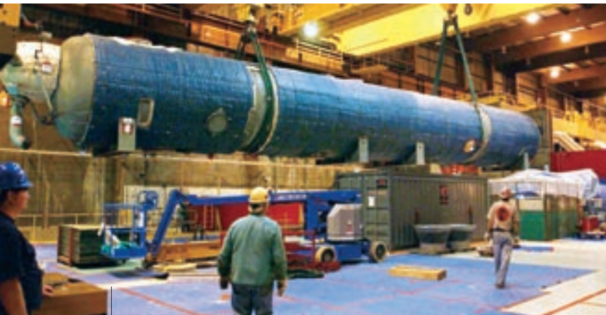
An MSR vessel is carefully transported across the turbine building floor during replacement.
