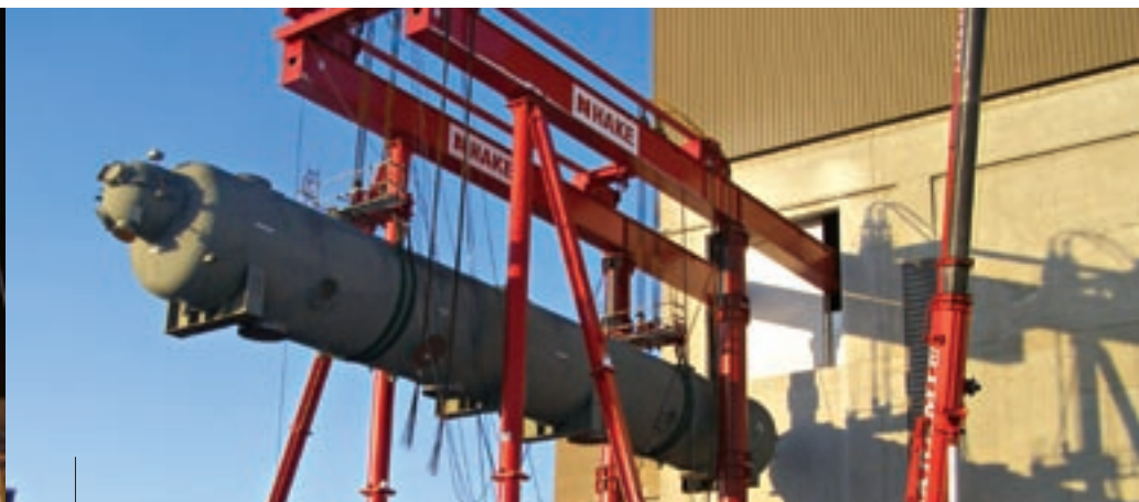
Using the modular lift tower, one of the two new 300-ton MSRs is lifted for installation during URS' retrofit of the plant.
