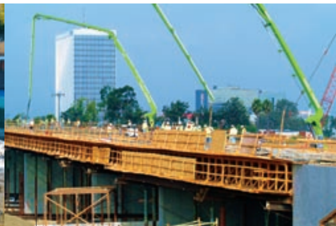
To increase the pace of construction, multiple concrete pumping machines simultaneously placed large quantities of concrete.
