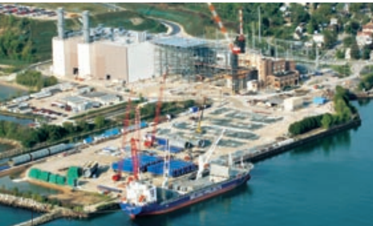
The plant's location on the shores of Lake Michigan enabled URS to have freighters deliver large components directly to the construction site.
