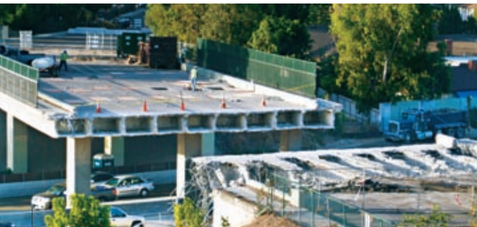
The Lewis Street Bridge over SR-22 was completely demolished and replaced with a new structure.
