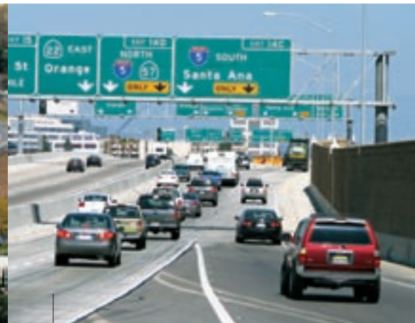
A concrete barrier was added to separate eastbound SR-22 traffic from traffic exiting to southbound Interstate 5.
