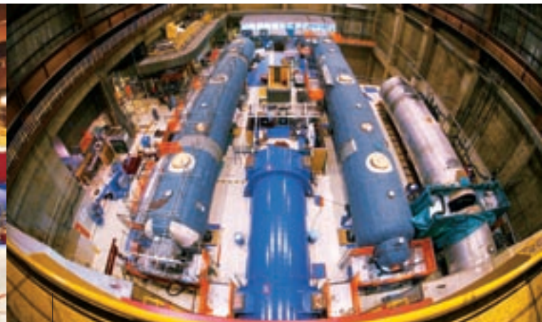
New one-piece MSRs are staged for installation on the turbine deck of the power plant, while one of the old two-piece vessels sits to the right during its removal.
