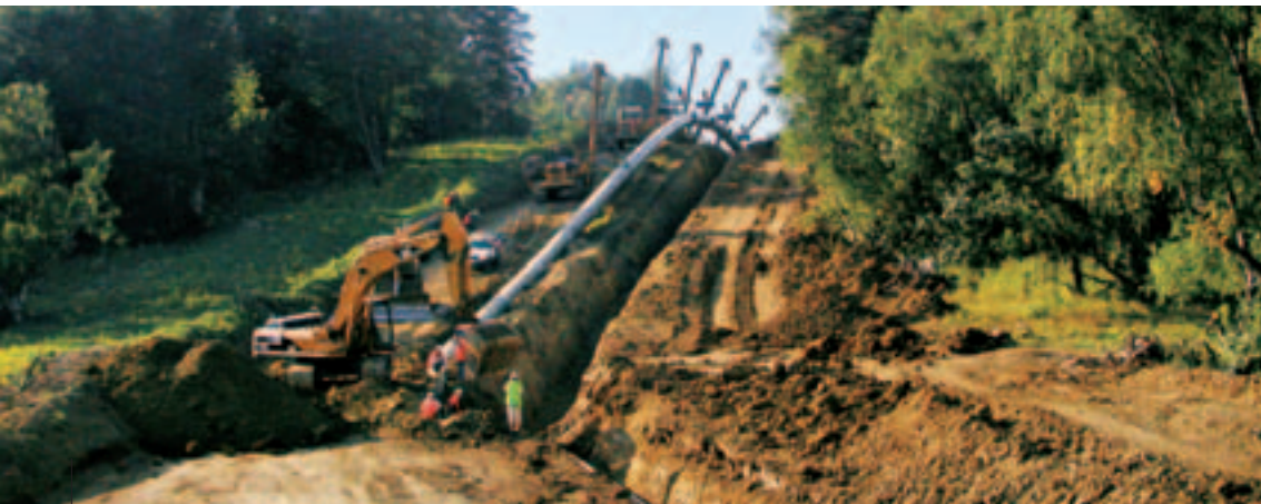
URS supervised the environmental aspects of the construction of a new BP pipeline through Georgia to Turkey.
