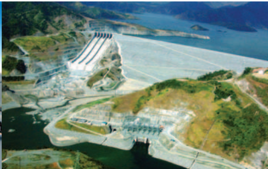
San Roque Power Corporation, San Roque Multipurpose Hydroelectric Project, Luzon, Philippines
