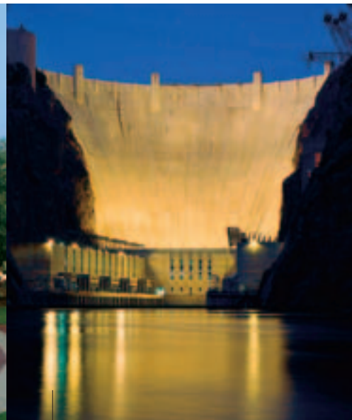
Hoover Dam across the Colorado River, Nevada/Arizona
