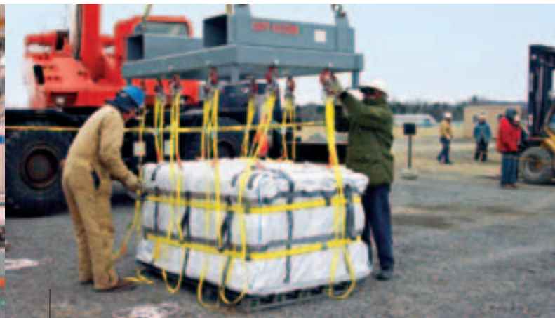
Low-level waste is prepared for transportation off site.
