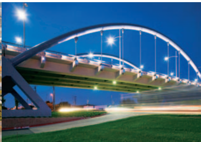
Arapahoe Arch Span Bridge, Addison, Texas
