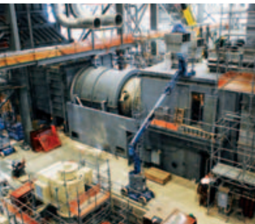
The gas-turbine enclosure incorporates various noise-attenuation features to limit the impact of operations on local residents.
