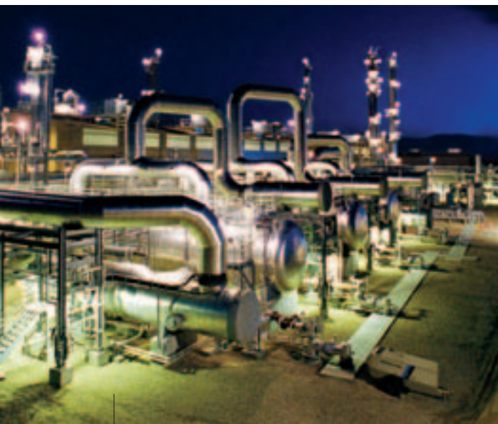
Lost Cabin Gas Processing Plant, ConocoPhillips, Lysite, Wyoming
