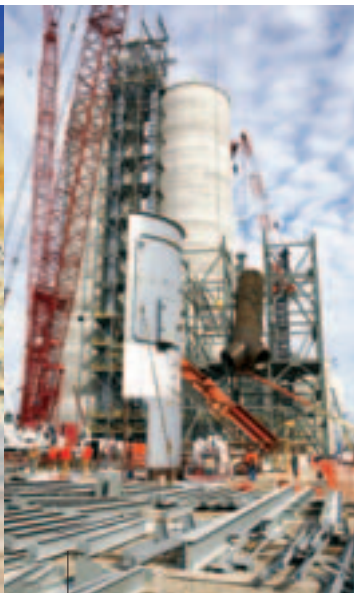
Holcim (US) Inc., Cement Manufacturing Complex, Ste. Genevieve County, Missouri
