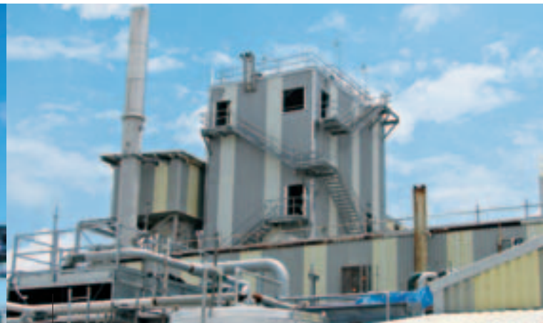
The retrofit of an existing plant required removing a freight elevator and performing major foundation work without disrupting plant operations.
