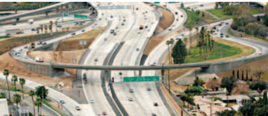
The Horseshoe Bridge provides a traffic connection for eastbound SR-22 to northbound Interstate 5 and SR-57.
