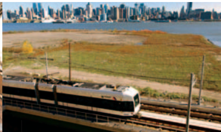
The Hudson-Bergen LRT system was honored with a Best of 2006 Award by New York Construction magazine.
