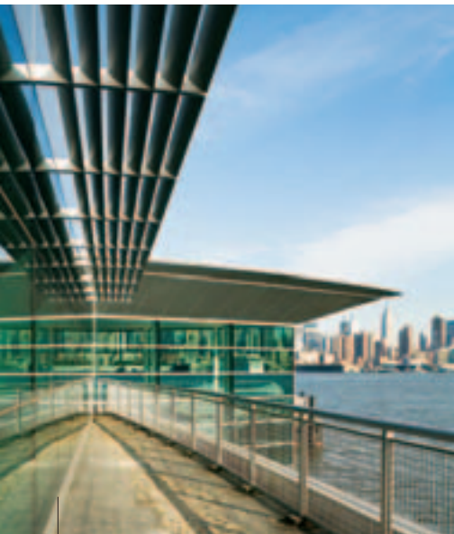
Port Imperial Ferry Terminal, Weehawken, New Jersey
