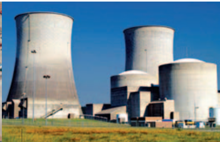
URS performed construction and start-up support for TVA's Watts Bar Nuclear Plant in Tennessee—the last new nuclear plant to go online in the United States.
