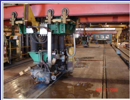
Automatic wet grinding of a plate before assembly
