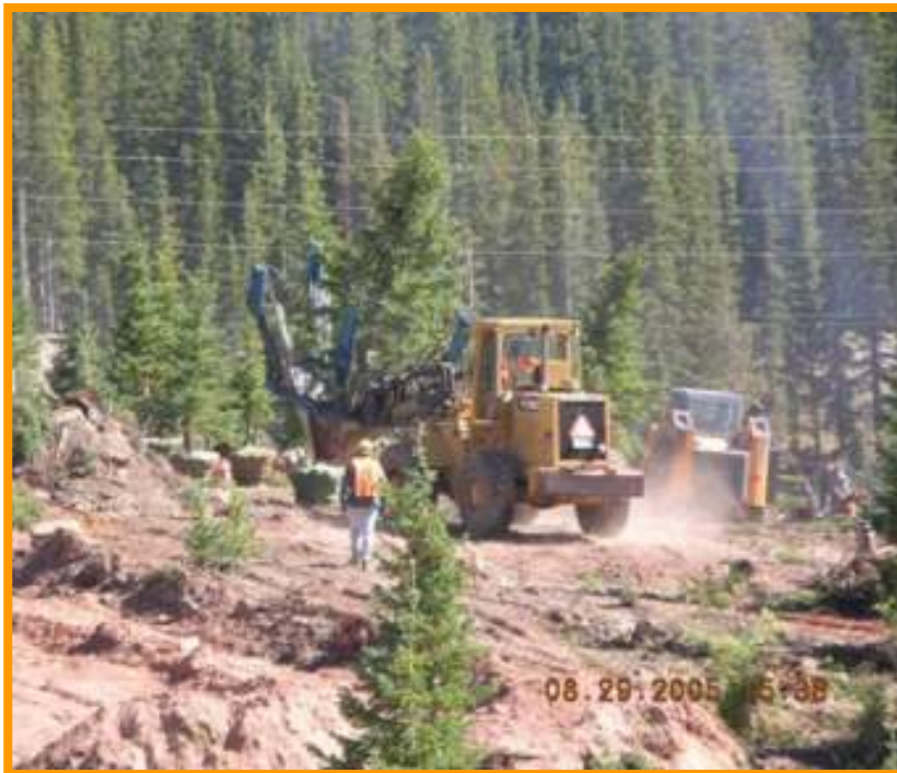
Tree removal at Tenmile Tailing Pond
