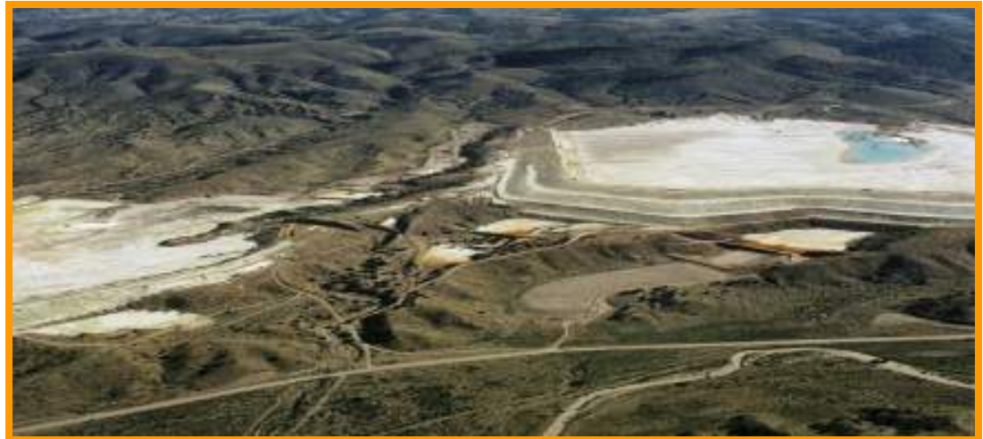
Tyrone Tailing Dam
