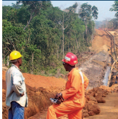
▶ The high profile Chad-Cameroon Pipeline project demonstrated Willbros' world-class capabilities.
