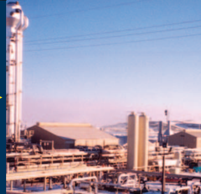
▶ Opal turbo-expander plant, a design, build and own project of Willbros Mt. West, was operating in early 2004.
