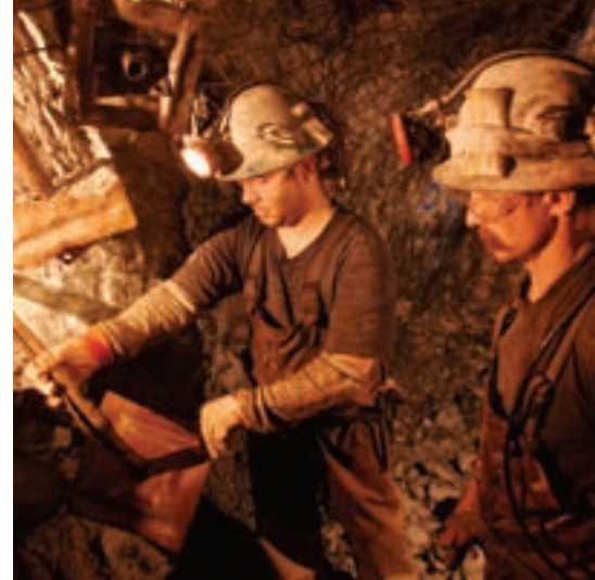
Preparing ground support.
