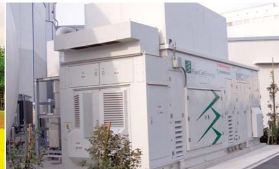
Tokyo Super Eco Town, Tokyo, Japan Our DFC power plant provides renewable base load electricity using biogas produced from food waste.
